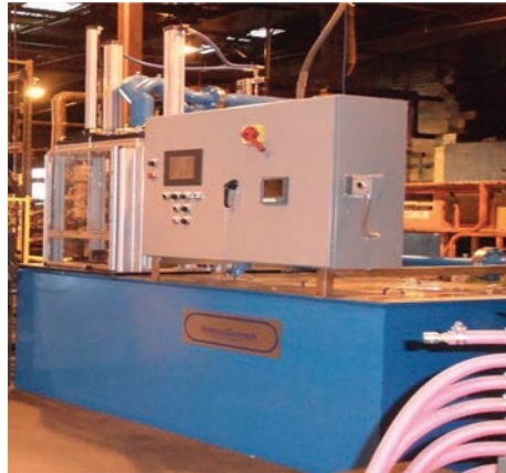
Fig. 22 Single-part processing IQ system installation at the IQ Technologies Center at Euclid Heat Treating Co.
